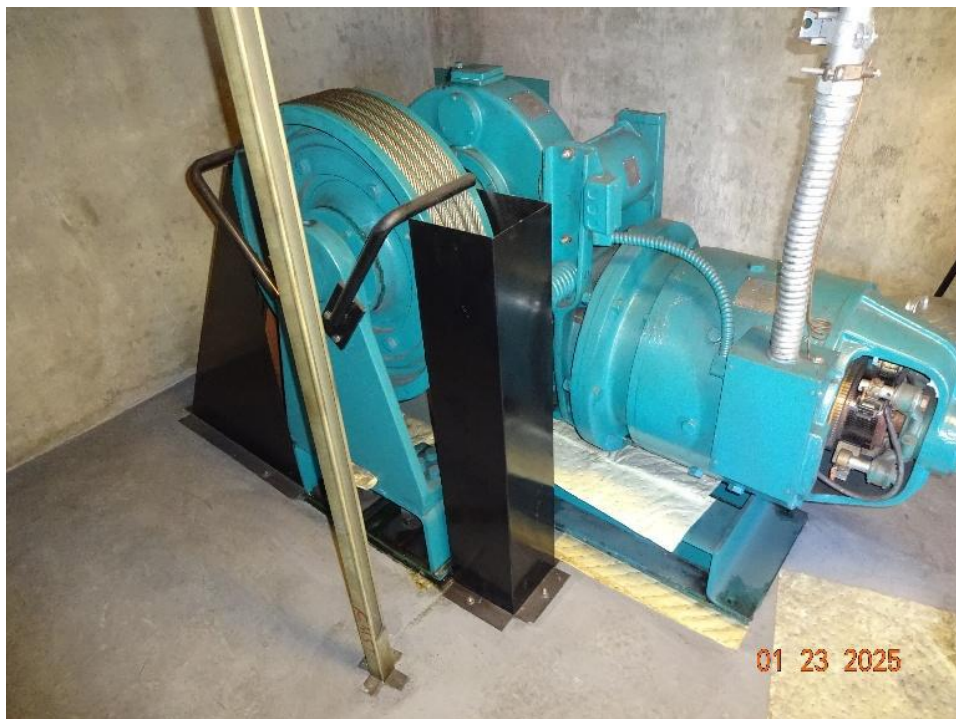
Existing outdated machine with DC motor drive to be replaced with modern AC drive
