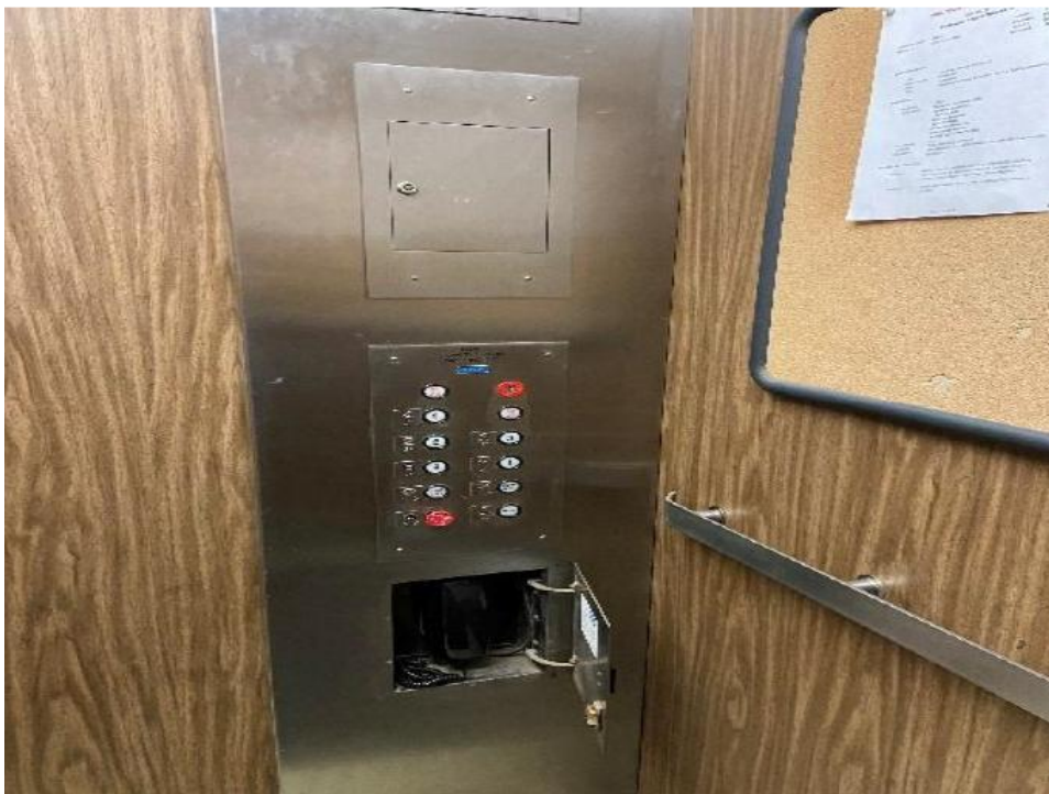
Existing outdated floor buttons to be updated to comply with modern code requirements
