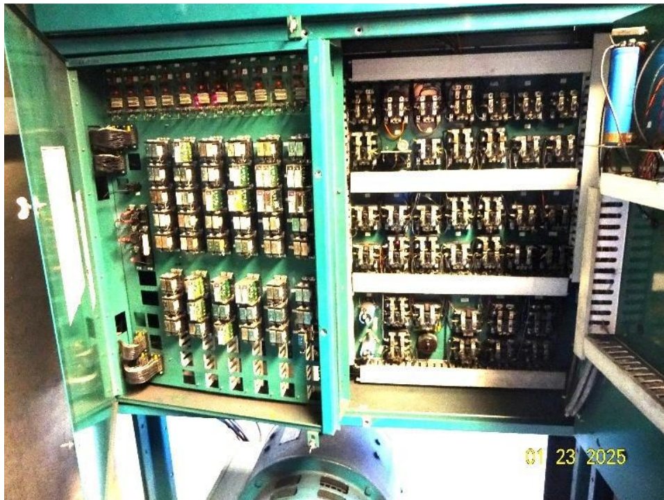
Existing outdated wire contact relay controller to be replaced with modern microprocessor
