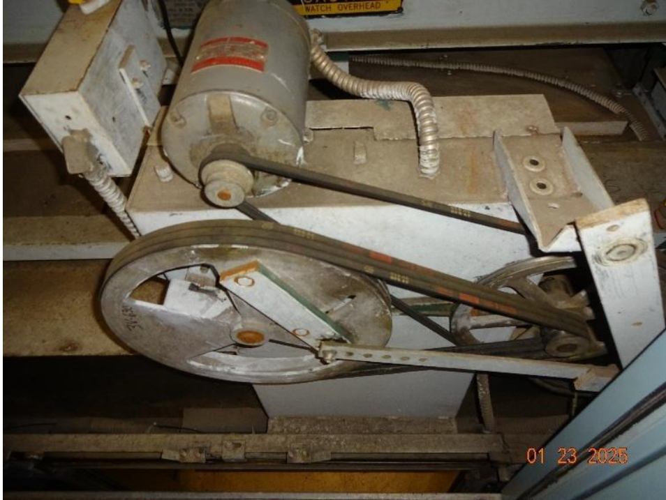
Existing outdated door operator to be replaced with a modern closed loop door operator
